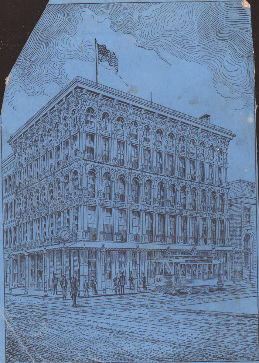
THE SUN BUILDING. SOUTH-EAST CORNER BALTIMORE AND SOUTH STREETS, BALTIMORE MD
